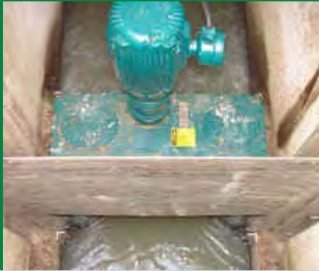
An immersible motor ® installed on a Channel Monster ® in a deep channel.
