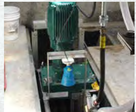
An immersible motor powers an Auger Monster ® in an underground vault.
