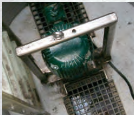
A Muffin Monster ® with immersible motor and lifting bail in a deep wet well.
