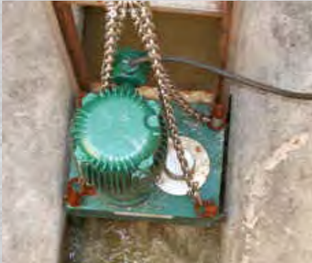
An overhead view of an immersible motor in a deep wet well.
